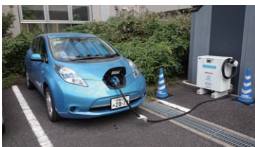
Vehicle to Building の実証実験
